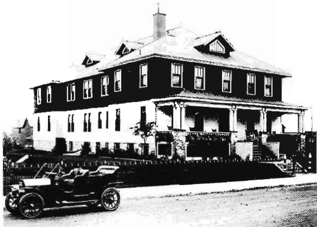
THE OLIVER Company clubhouse in Hibbing as it looked about 1910
