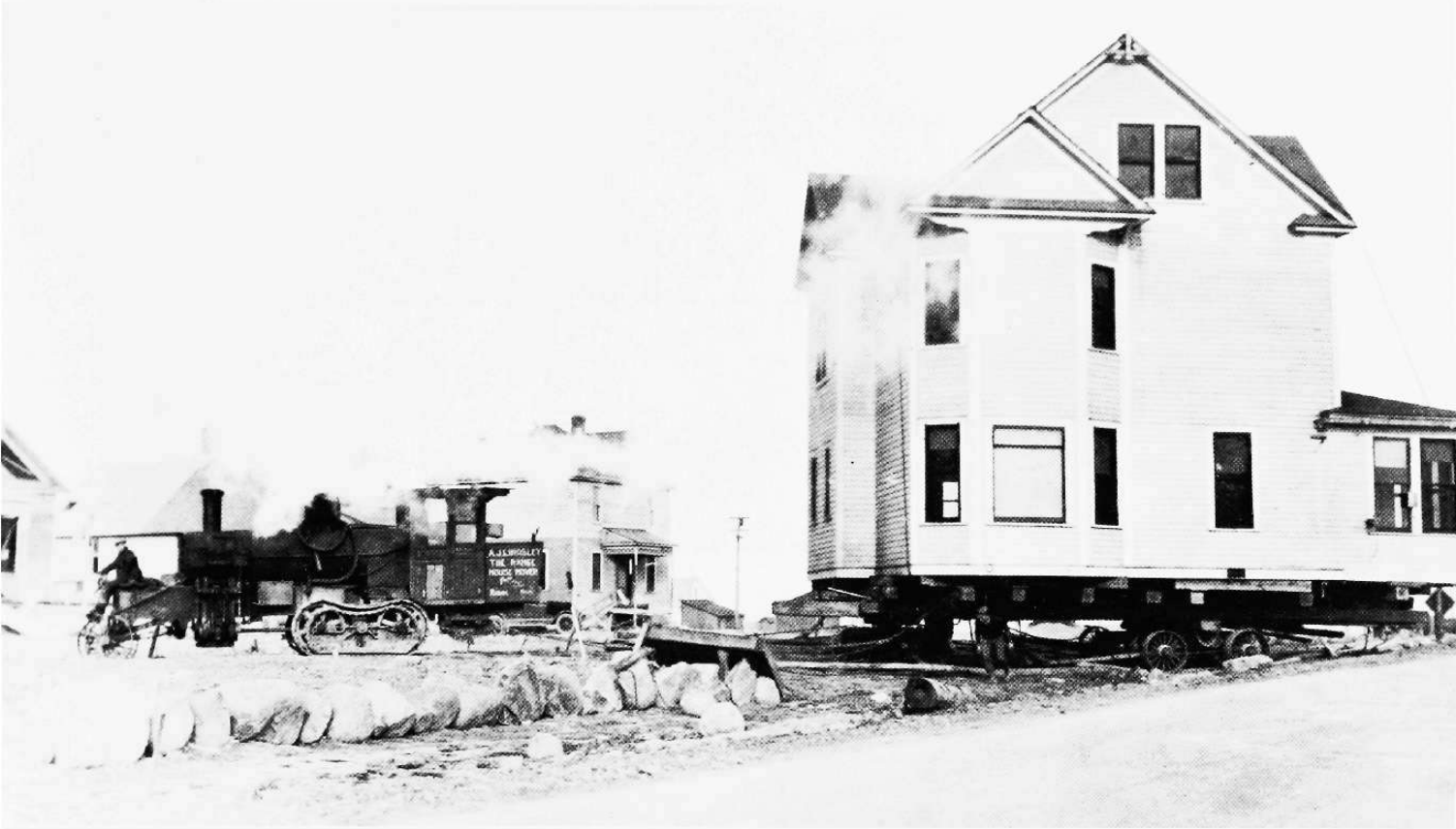
"THE RANGE House Mover," A. J. Lindsley, pulling one of the better-built location houses to a new area
